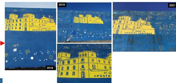
The **color deterioration** of the base blue paint is very clear in these images: a color protector was applied in the area of the square in 2018. In 2021, the unprotected blue paint lost its color whereas the protected area remained unaltered. Note the intense **delamination** affecting blue base paint.
